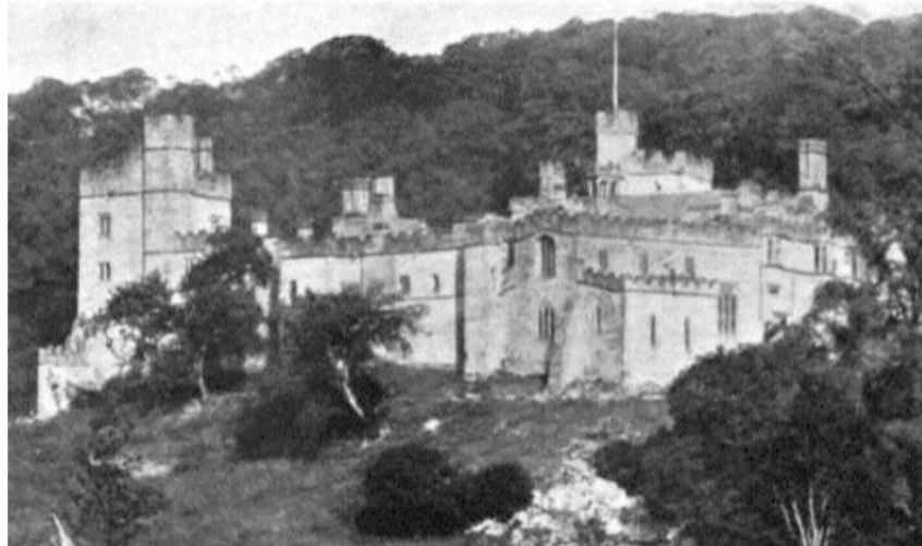
[Haddon Hall, West Face]
